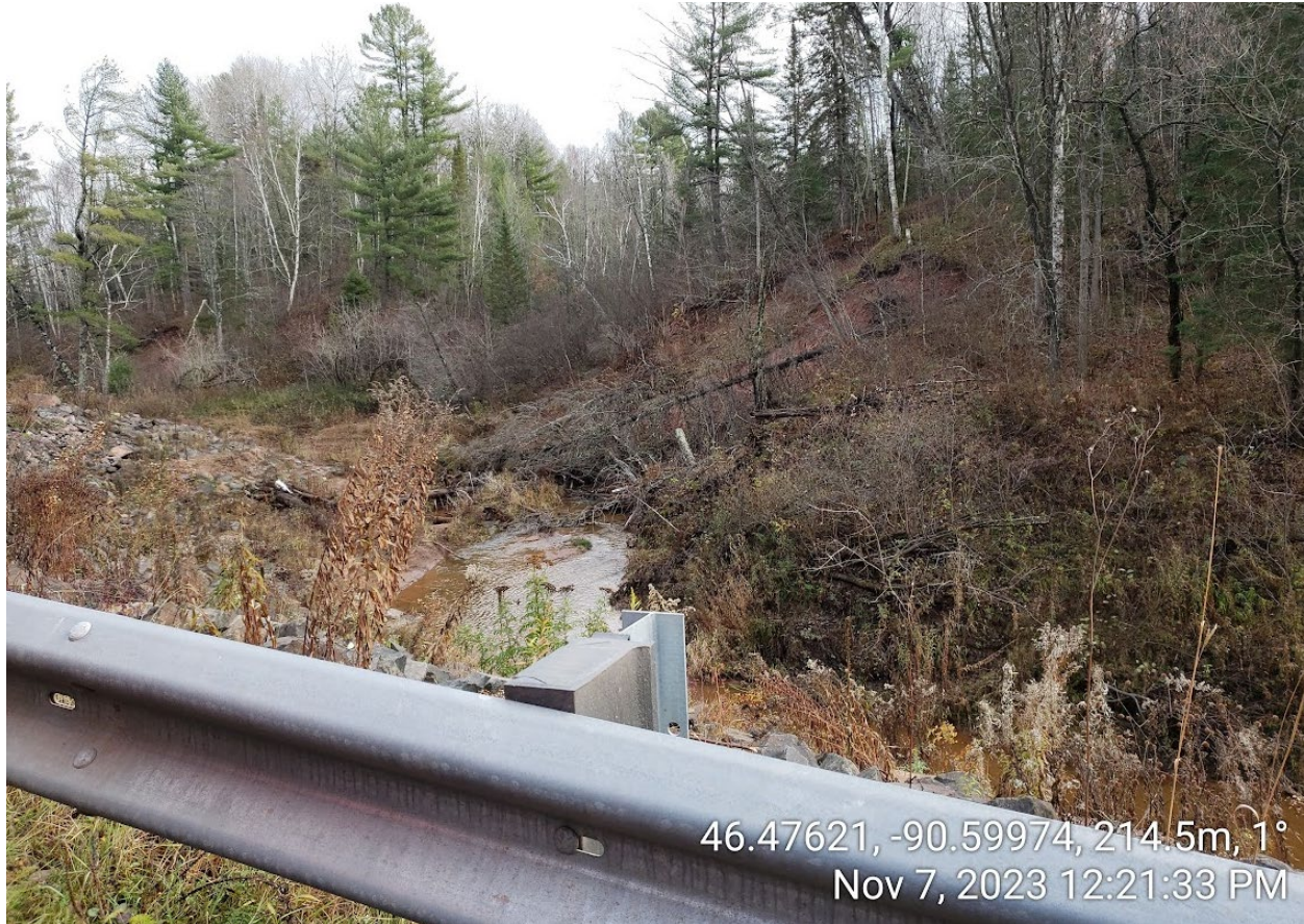
Figure 5. Winks Creek as it flows from the washout in 2023, seven years after the storms that contributed to the mass wasting failure at the road and erosion still apparent on the banks downstream.
