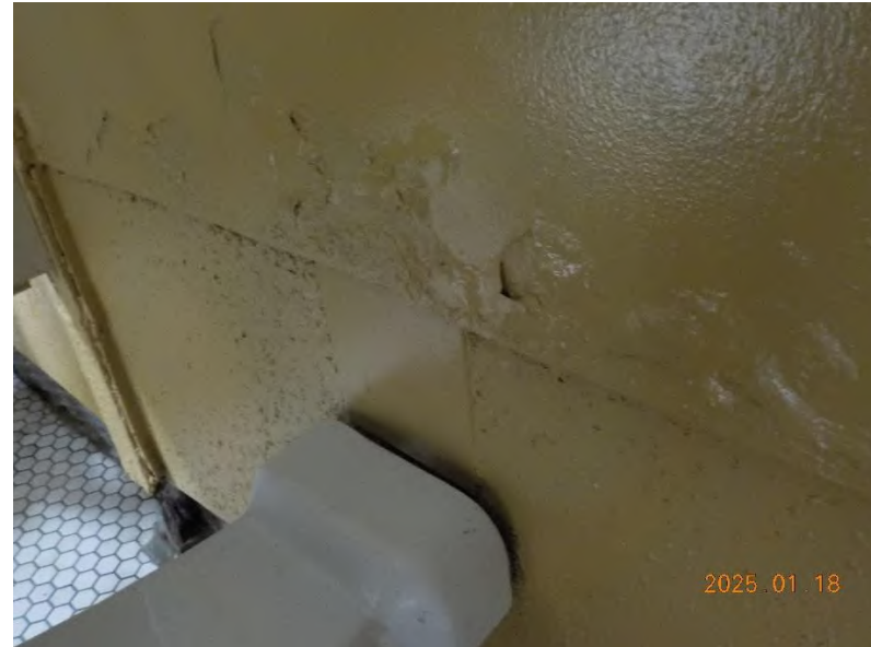
Boy's bathroom wall C (south) along toilet stalls (stall #6 shown)
