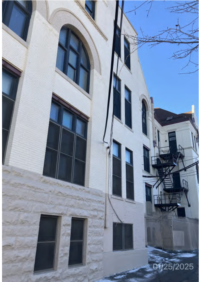
Exterior side C
